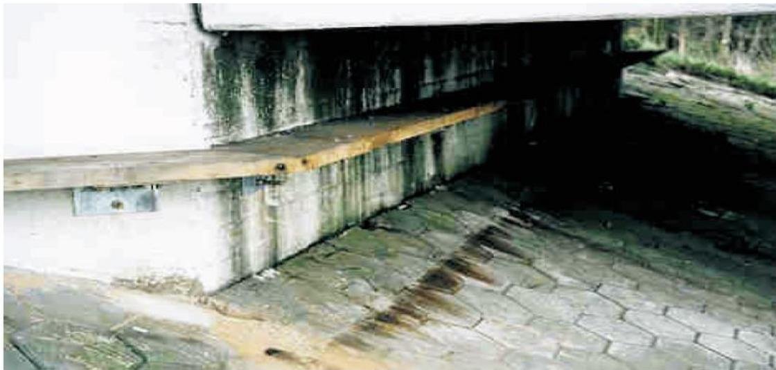
**Illustration 5:** Water conduit with a ledge enabling wildlife traffic even when the passage is flooded.
