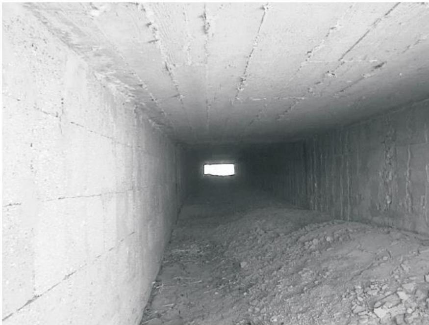
**Illustration 6:** A water conduit half-blocked by earth and gravel.
